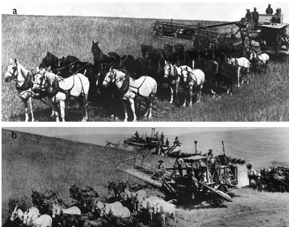
Fig. 12. (a) The ground-driven, horse-drawn combine replaced the station-ary thresher (see Fig. 5b) in earnest about 1910. The larger machines with 6-m headers required a four- to six-man crew and 27 to 34 horses or mules. Straw was spread on the ground and grain was sacked and piled into small stacks of four or five sacks in the field before hauling to ware-houses. Photo from Brumfield (1968). (b) Gasoline engines began to replace the ground-drive combine in the late teens that reduced manpower re-quirements and horses by about one-third. Photo from Northwest Museum of Arts and Culture, Spokane, WA, L93-62.10.
