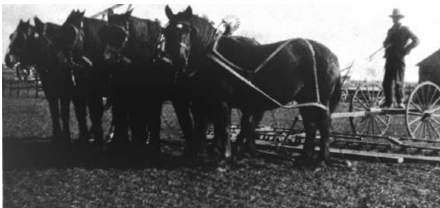
Fig. 7. The spike-tooth harrow was commonly used to control weeds in summer fallow before the advent of the rotating rodweeder (see Fig. 10). Most early farmers thought it was necessary to pulverize the surface soil to maintain soil water during summer fallow. Those who pulverized the surface soil were considered good farmers. The combination of primary spring tillage with a moldboard plow followed by repeated harrowing operations to create a soil surface devoid of residue, clods, and roughness led to massive and recurrent wind erosion. Photo from Adams County Historical Society (1986b).
