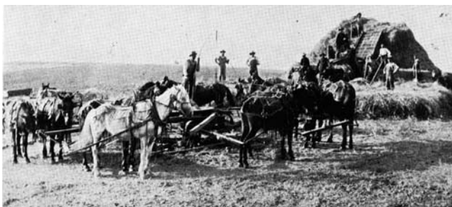
Fig. 4. An early stationary grain thresher powered by 12 horses. Note the conveyor system at the back of the thresher for elevating straw to the top of the pile. Steam engines had almost completely replaced horses to power threshing machines by the turn of the century. Photo from Brumfield (1968).
